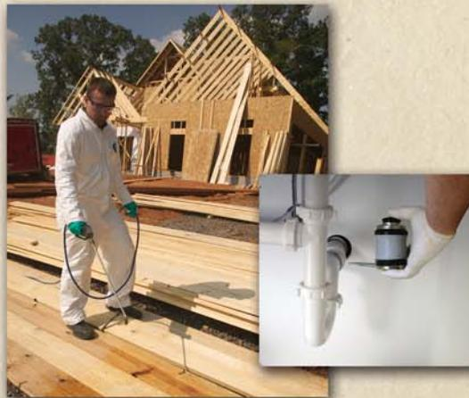
Tim-bor Professional's active ingredient is a natural borate mineral salt that diffuses into wood and will not break down over time like most organic compounds.
